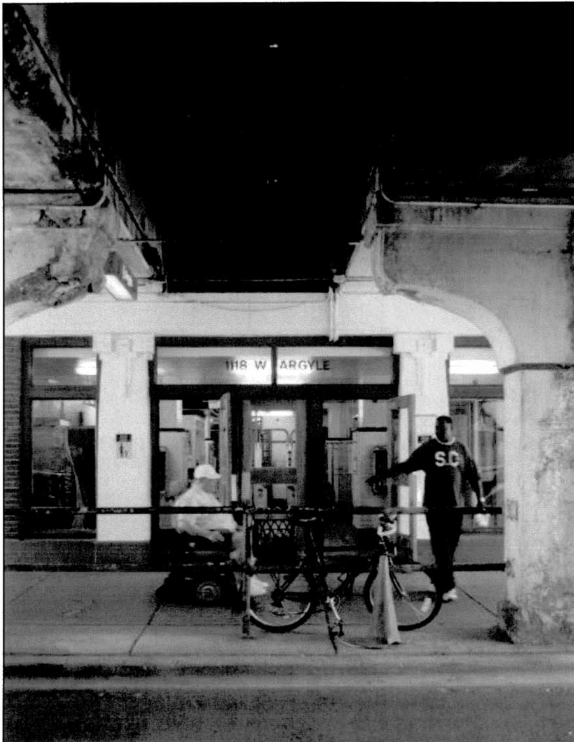
West Argyle Street station for elevated rail (1922)
